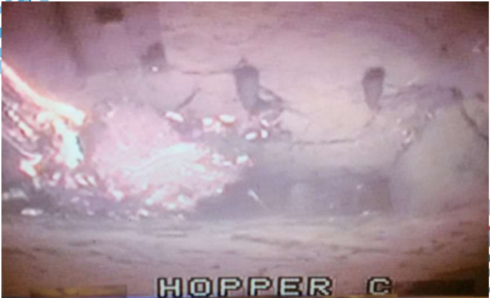
Live Camera Shot from inside “Hopper C” of the new dry bottom ash hopper.
